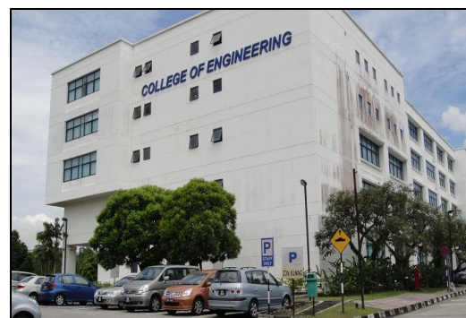
Fig.3: BN Building in COE
